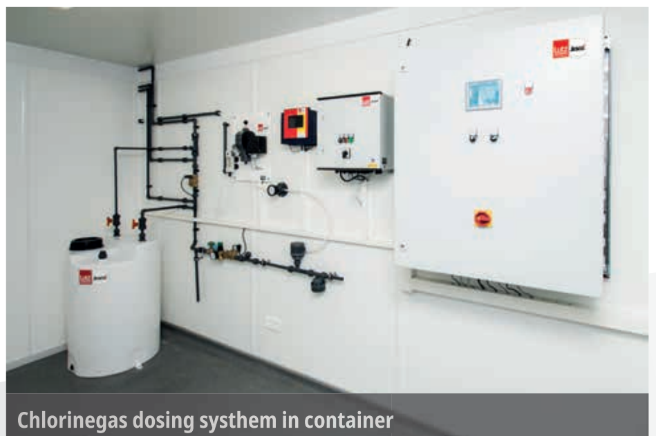
Plate-fitted dosing system in a weather-protected cabinet
