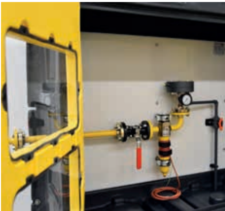
Plate-fitted dosing system in a weather-protected cabinet
