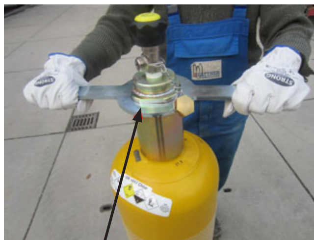
Fig. 2: Tightening the emergency cap with the special wrench
